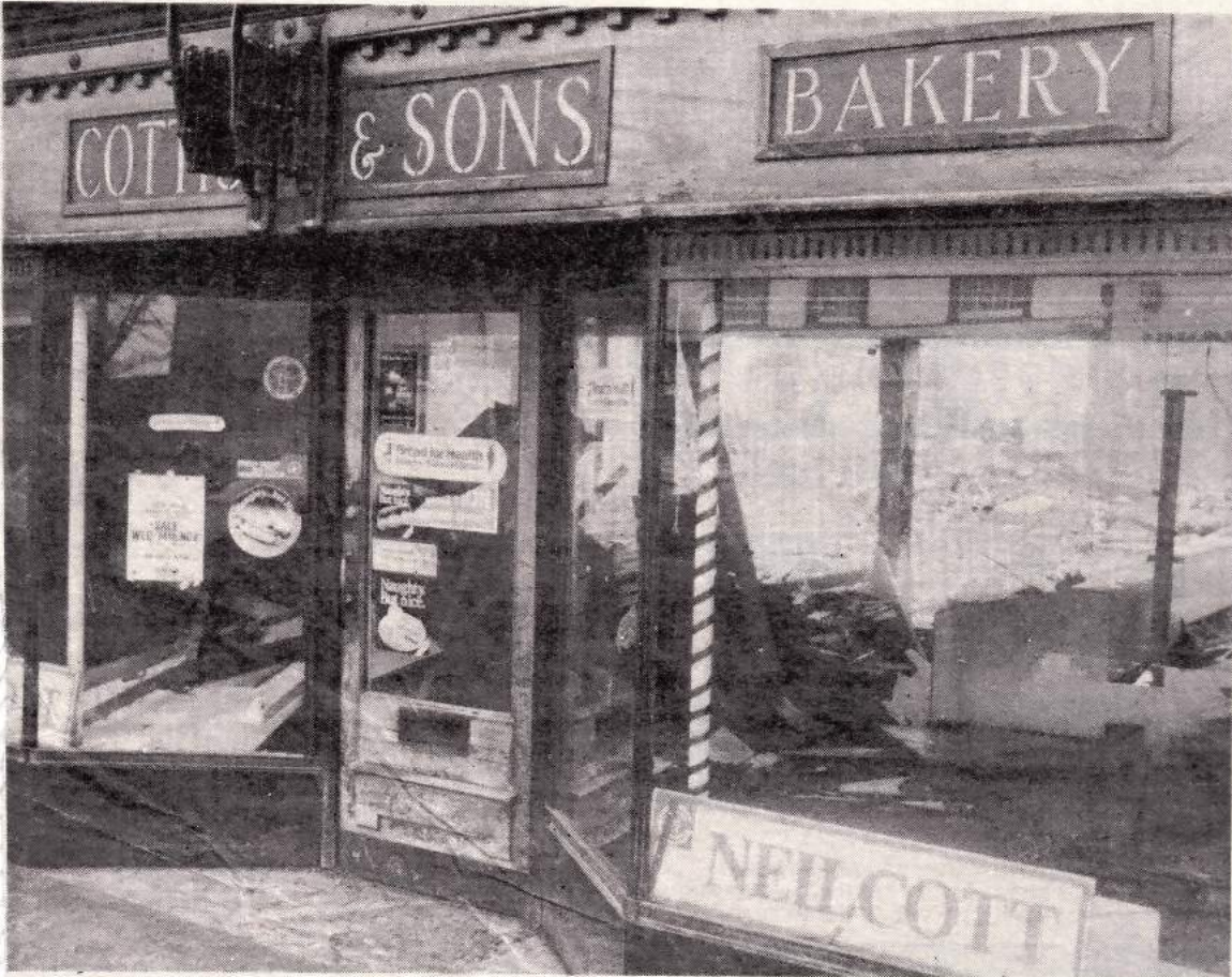
Demolition work at the former Cottis bakery.
